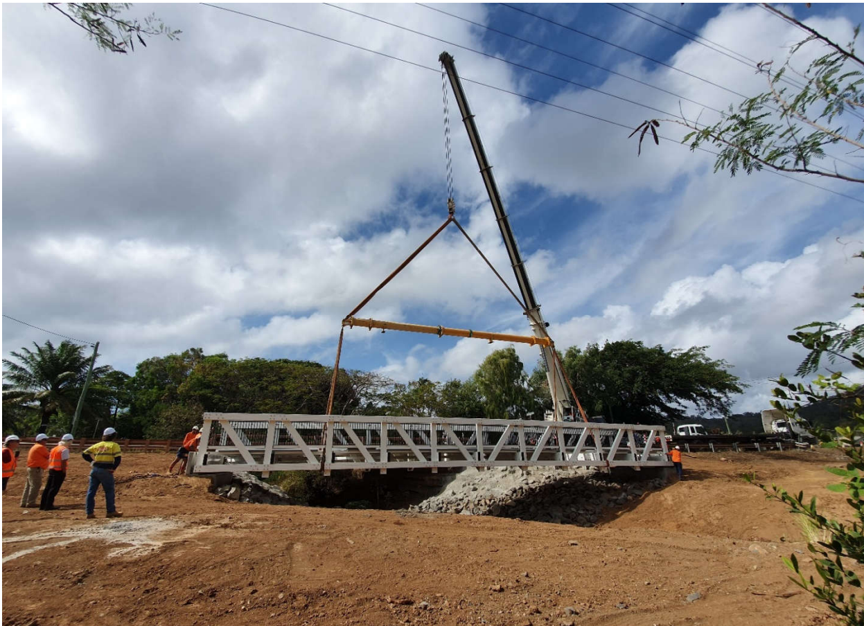
Cycle/Footpath at Two Mile Creek Bridge Construction
